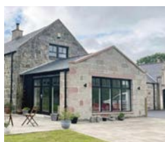
Extension with Internal Alterations
