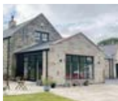
Extension with Internal Alterations
