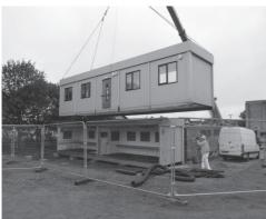
Cabins being craned in... thanks to Greenwell for supplying the cabins (ex-classroom in Oban) and Global Port Services for the crane
